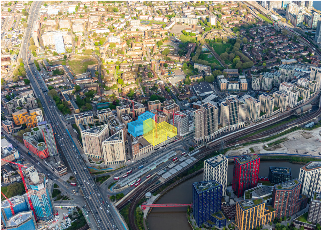
Image taken: 07/05/2023 – shaded buildings now completed. The subject property forms part ground floor of the building shaded blue.
